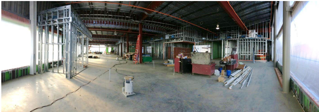
Project Site on November 27, 2019 Interior Panoramic View from the Sherman Entrance.
