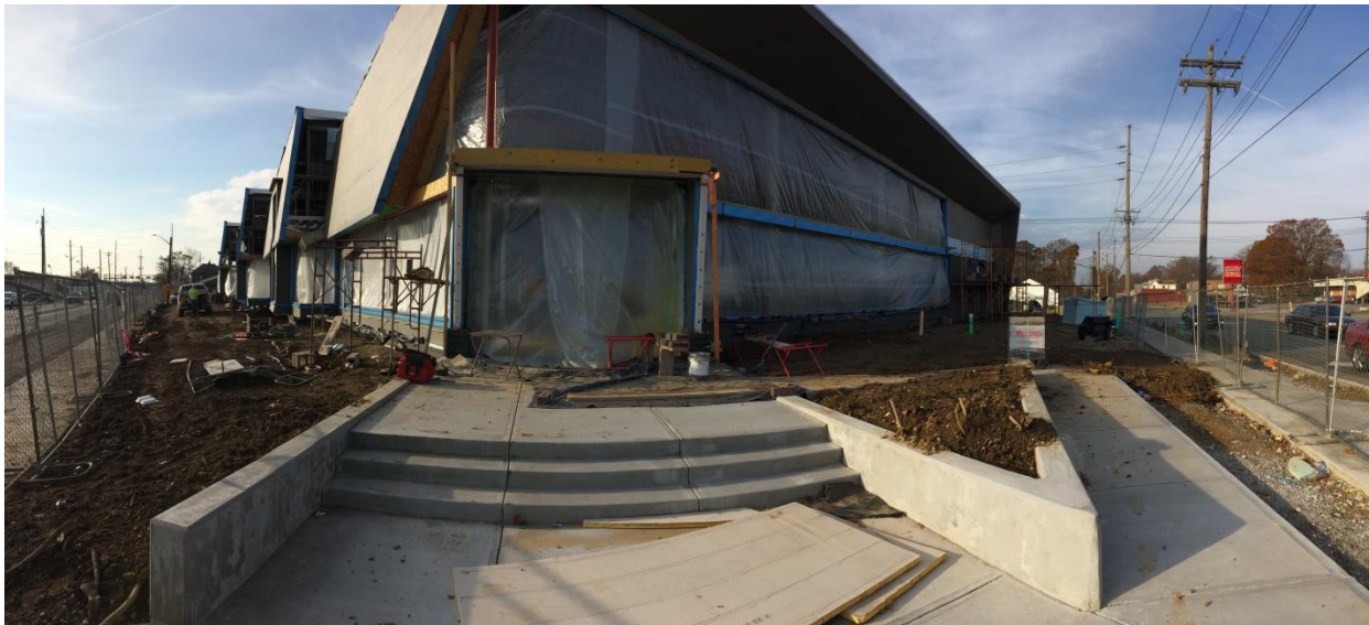
Project Site on November 27, 2019
