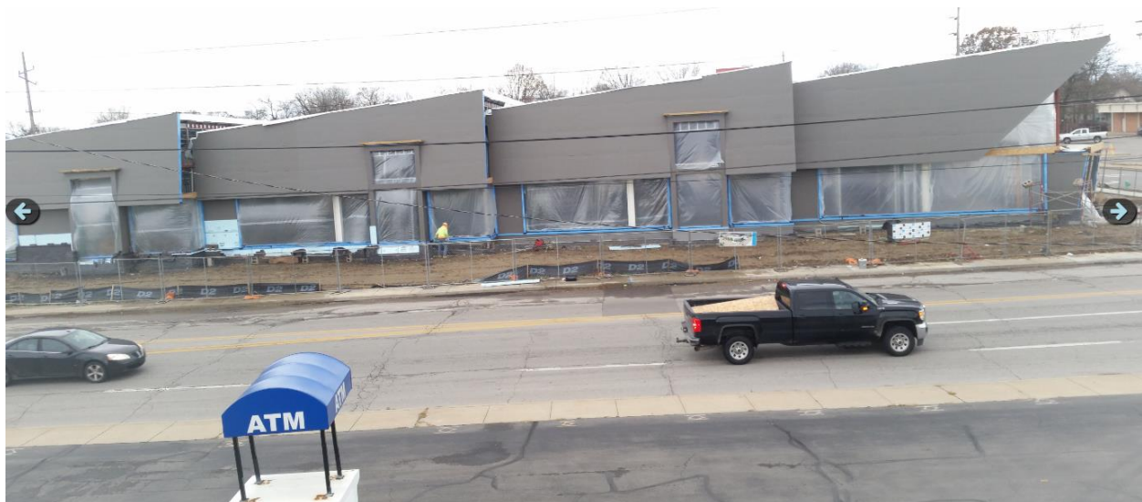
Project Site on November 27, 2019
